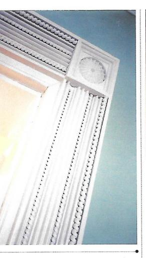
Element of Surprise: Concealed under countless layers of paint applied over the last two centuries, some of the home's original intricate mouldings, like those on this interior door frame, were uncovered during restoration.
